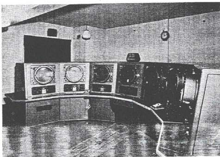
The seven 15 in. display units at Gladstone Dock
